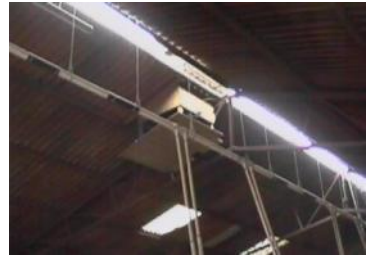
Condition of vents
